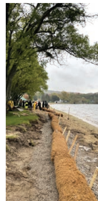
Positioning coir logs before finalizing installation. Photo: J. Kirkwood
