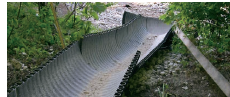
Photo depicting a rock chute to transport rocks to reduce impact. Photo: J. Buchanan
