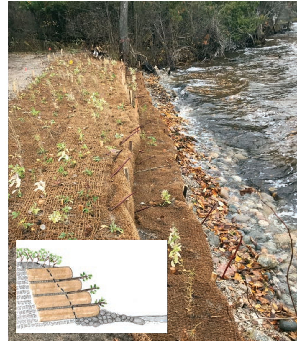
Figure 9: An encapsulated soil lift design and installation. Photo: TOMWC
