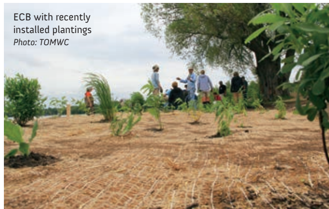
Contractors beginning installation of ECB. Photo: J. Buchanan
