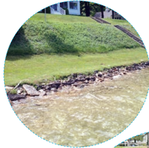
Receding shoreline: Example where the addition of rock is ineffective due to improper design and lack of shoreline vegetation.
