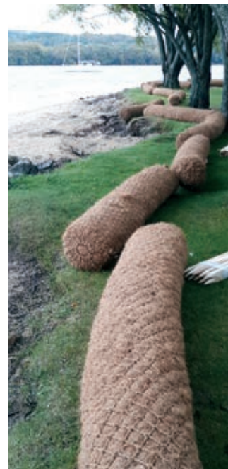
Coir logs staged along shoreline prior to installation. Photo: J. Buchanan
